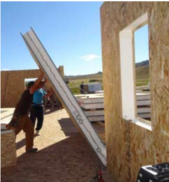
IMAGE 7.4 SIP WALL SEALANT APPLICATION
