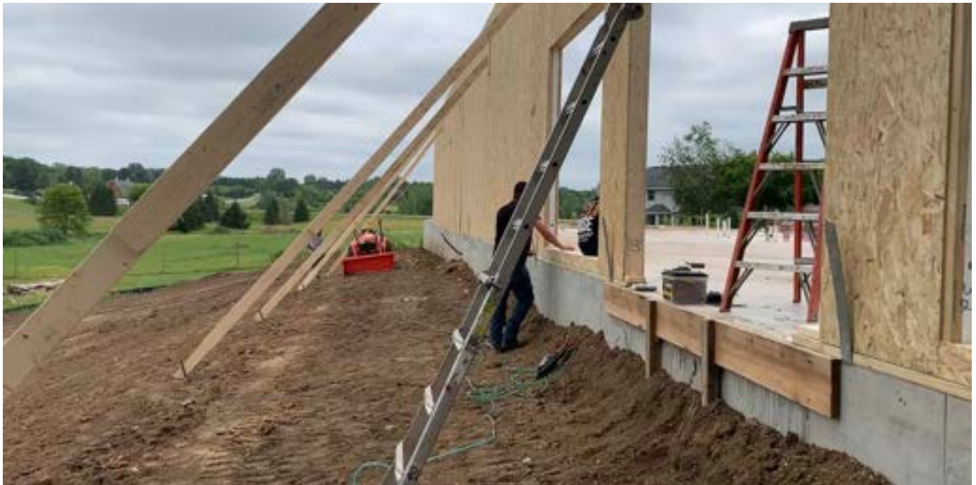
IMAGE 7.28 EXTERIOR SIP WALL BRACING FROM THE EXTERIOR OF THE BUILDING
