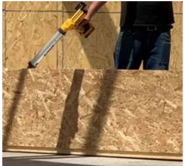
IMAGE 7.3 AUTOMATED SEALANT APPLICATOR
