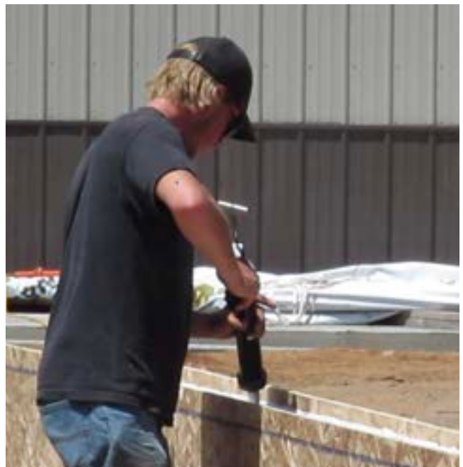
IMAGE 7.5 SIP WALL SEALANT WITH MANUAL APPLICATOR
