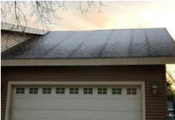
IMAGE 1.3: SIP GARAGE ROOF
