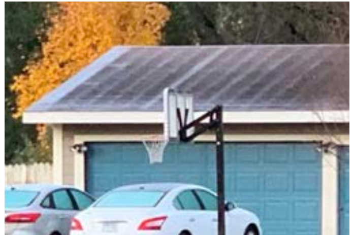
IMAGE 1.4: TRADITIONAL GARAGE ROOF
