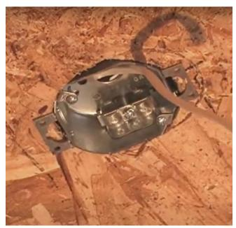
Note: not shown are the four screw fasteners required to support the weight of a ceiling fan.
